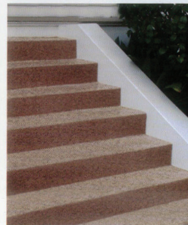
Installed with Tile Texture Roller
